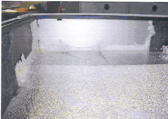
Back side and edges with silicone sealed
