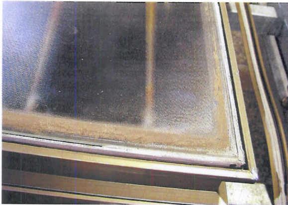
Connection frame/glass with silicone
