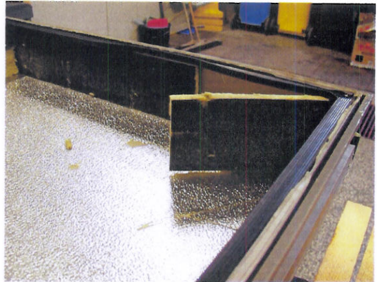
Bonded 10 mm of side wall insulation
