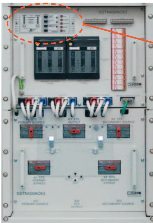
Static Transfer Switch SSTN400AC63 rack
