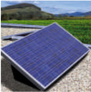
Fast, flexible and uncomplicated: assembly of the ConSole 4.2.
