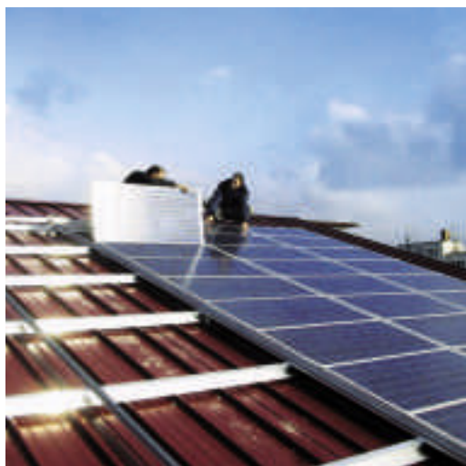
Unique case: a double-layer IBC MEGALINE STANDARD slanting roof mount being installed on a trapezoidal roof.
